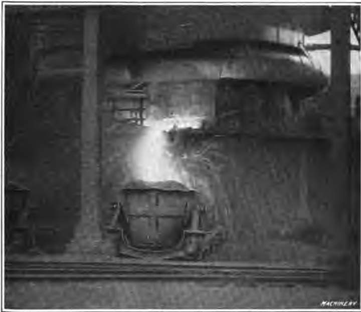
Fig. 4. Ladle receiving Molten Metal from Blast Furnace
